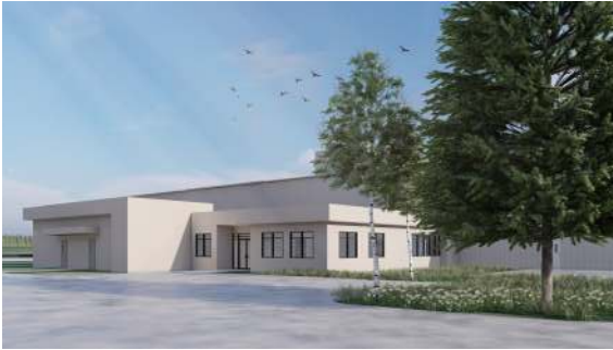
MAIN OFFICE BUILDING - EAST VIEWPOINT
