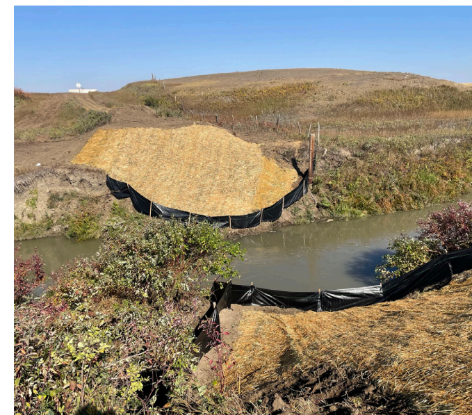
BF 13884 - Bridge Removal
