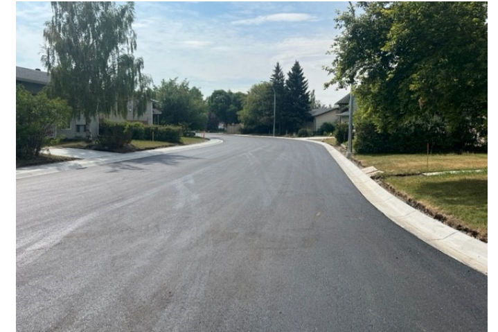
Carseland - Cole Crescent Sanitary Line Repairs and Pavement Replacement
