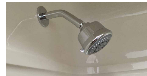
Newly installed low-flow shower head in a resident's home
